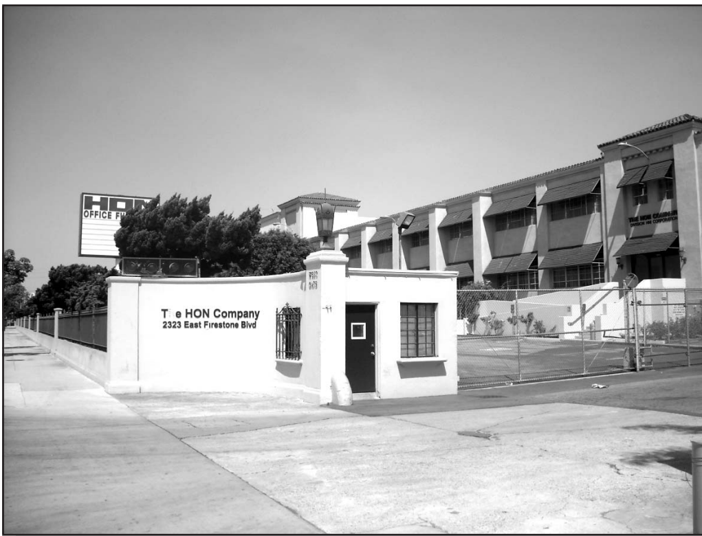
View of the south-facing facade of Buildings 1 and 2 located on the western project site from Firestone Boulevard.
